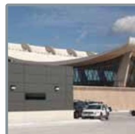
Washington Dulles International Airport (IAD) Chantilly, VA
